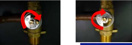
**Note:** the brass tab does not move; the round stainless steel cover plate with "IN" and "OUT" indicated rotates; the brass tab is part of the casting and is fixed;
